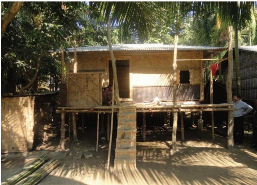
Figure 5 Photograph of a completed Machan House. (Credits: O. Moles et al.).
