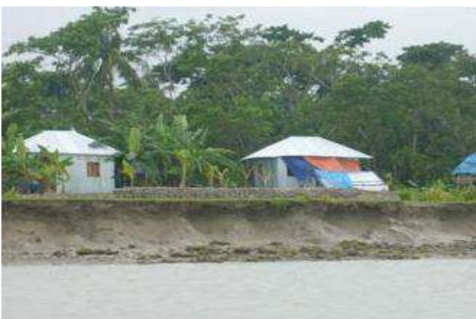
Figure 1. Construction of houses after the cyclone Sidr 2007.
