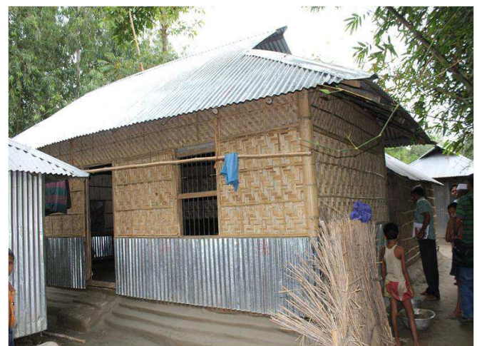
Figure 8. Photograph of completed house at Gaibandha. Main design considerations were to construct a house which can be dismantled within a short notice (based on local practice identified during the assessment of local practice). Also different types of 'katla' (which provides joint between the post and foundation) have been used to see their perfor-
