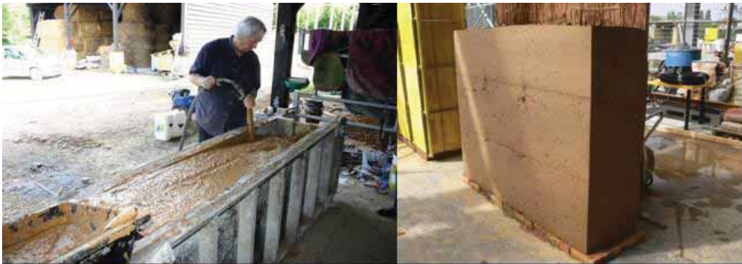
Fig. 5 - Poured earth and the obtained wall without cracks (© CRAterre-ENSAG)
