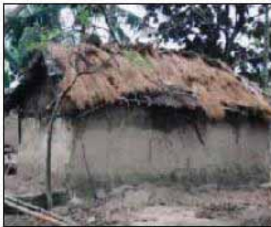
Fig. 7 - Mud House with Straw Roof
