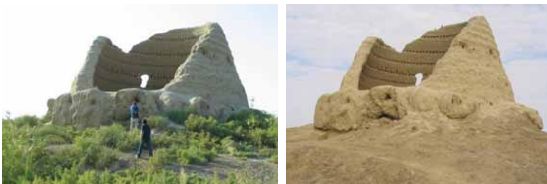
Fig. 1 - Ice House 2 – Removal of the plants on the building and its surroundings
