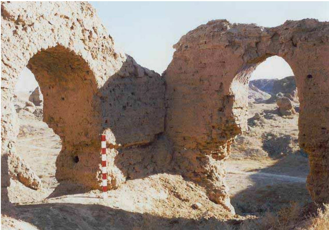
Fig. 5 - One of the Rooms in South of Kohan-dej that shows the Mud Brick Structure
