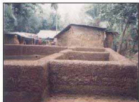
Fig. 12 - Mud Wall Construction
