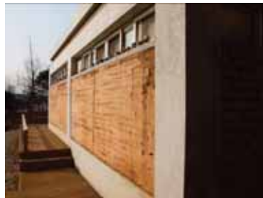
Building in pisé
