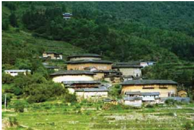
Fig. 4 - Earth buildings groups in Fujian Province
