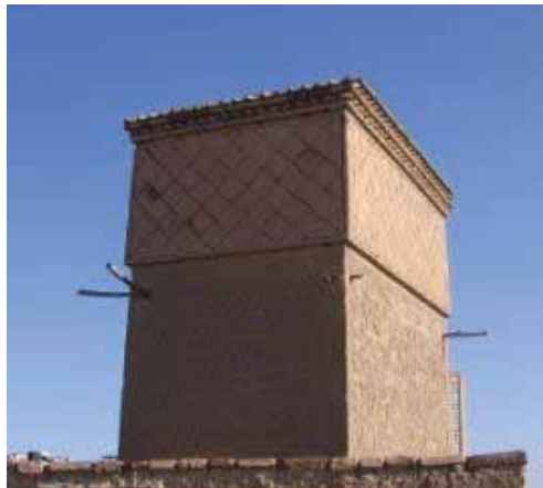
Fig. 6 - Stalk of a destroyed badgir in Sahlebneali quarter of Yazd (Authors)
