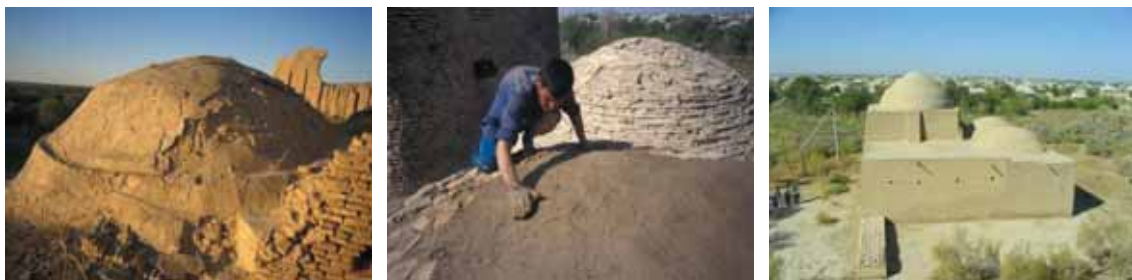
Fig. 3 - Ibn Zayd mausoleum – Sacrificial layers of mud mixtures are applied to protect the domed roof instead of the previous destructive cement coating
