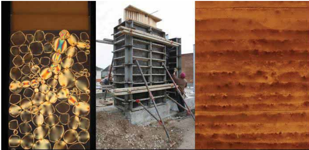
Fig. 1- In granular matter, stresses are transmitted through a network of forces chains, and usually deflected horizontally. That's why formworks must be very strong and rammed earth is compacted in thin layers (© CRAterre-ENSAG)
