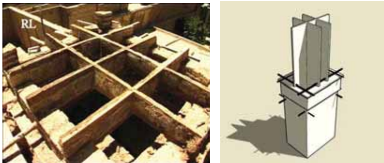
Fig. 7 - above left) : the major partitions of a constructing badgir
