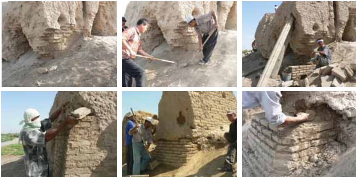
Fig. 5 - Reintegration of masonry at the corner of an eroded wall 2007
