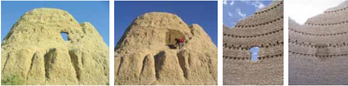
Fig. 6 - Ice house 2 - Reintegration of the masonry on the damaged dome in 2004
