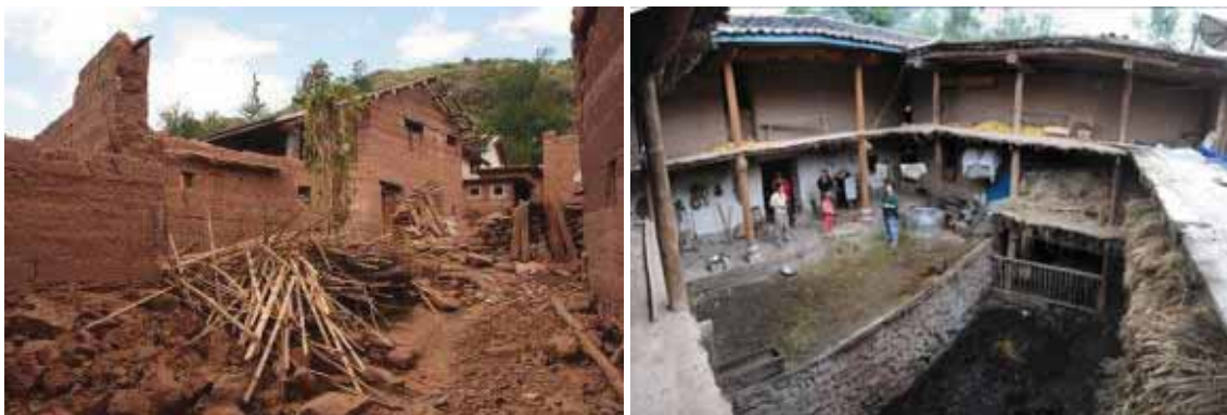
Fig. 2 - Local traditional rammed-earth courtyard dwellings and damaged houses after the earthquake
