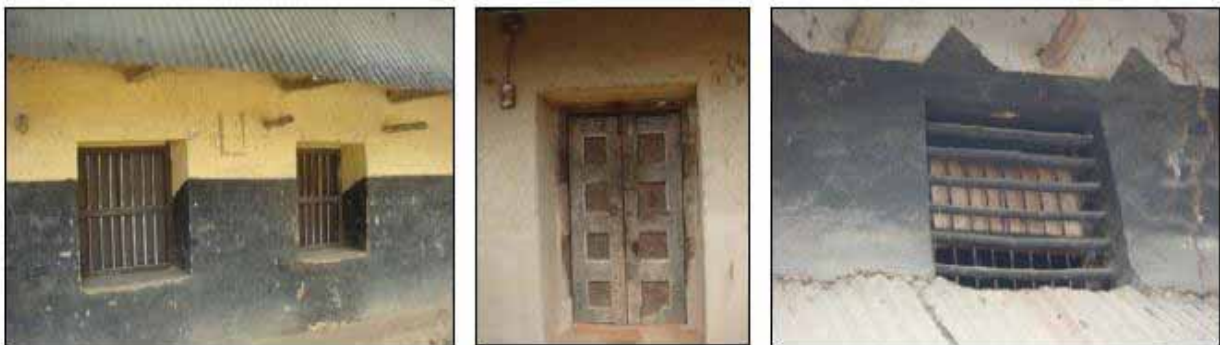
Fig. 14 - Settings of window (left), door (middle) and skylight (right)
