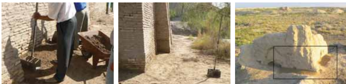
Fig. 4 - Peripheral drainage along the walls of Ibn Zayd mausoleum and Shahryar Ark palace
