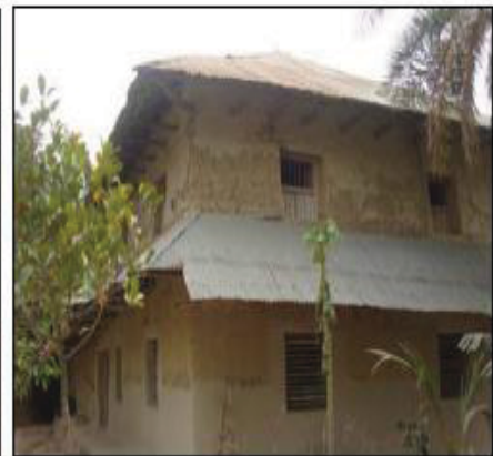
Fig. 6 - Double Storey Mud House
