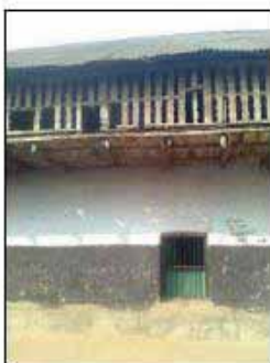
Fig. 10 - Palm tree in Ceiling & Balcony
