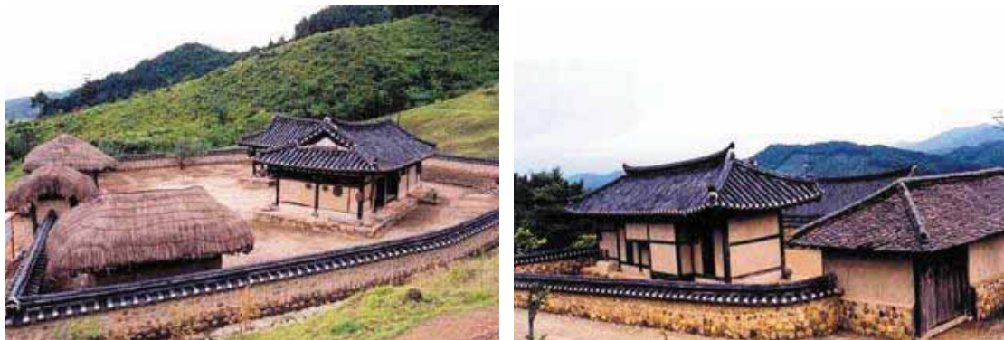
Fig. 1 & 2 - examples of Korean traditional houses; Hanyok and Chogajob , which were built of earthen material with wooden structures (captured from the web page of the Cultural Heritage Administration of Korea).
