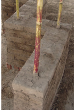
Peru vertical reinforcement paraseismic system
