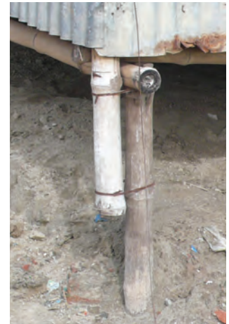
Bangladesh changeable pole-pile fixing flood-resistant system
