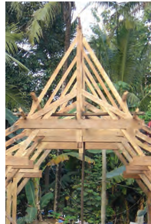
Indonesia wooden structure paraseismic system
