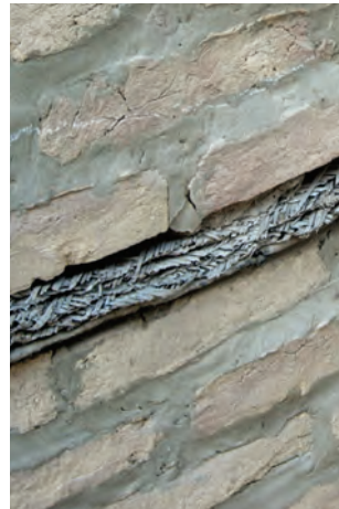
Uzbekistan reeds in adobe masonry paraseismic system
