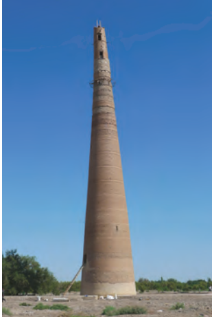
Turkmenistan frustoconical shape weak horizontal joints - strong vertical joints paraseismic system
