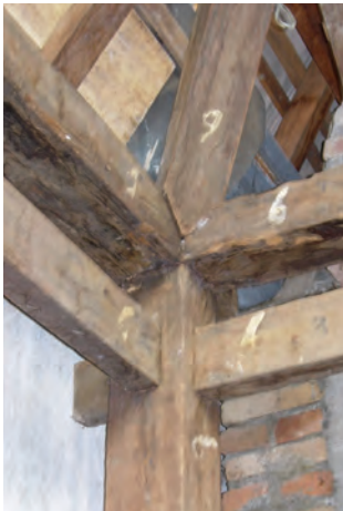
Indonesia post-frame connection paraseismic system
