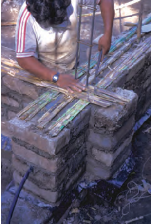
El Salvador horizontal reinforcement paraseismic system
