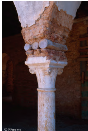
Algeria wooden rods on column paraseismic system
