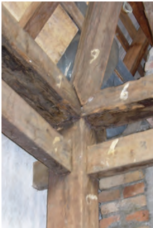
Indonesia post-frame connection paraseismic system
