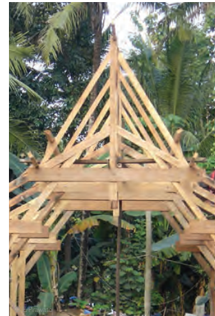
Indonesia wooden structure paraseismic system
