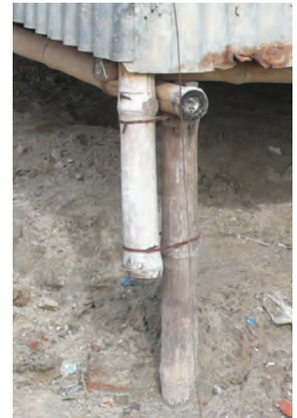
Bangladesh changeable pole-pile fixing flood-resistant system
