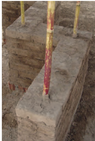
Peru vertical reinforcement paraseismic system
