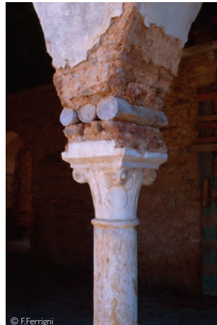
Algeria wooden rods on column paraseismic system
