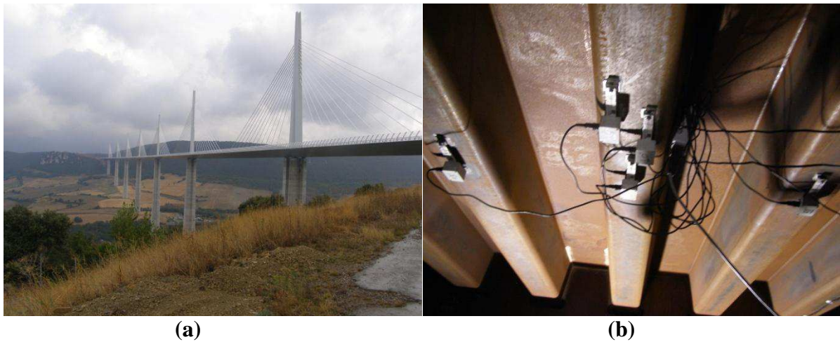
Figure 5: (a) Picture of the viaduct of Millau, with its 7 piers and pylon. The pier number 2, is the highest in the world with 245m. (b) Picture of the inside of the caisson with two extensometers used in the case of B-WIM adapted to metal bridges.
