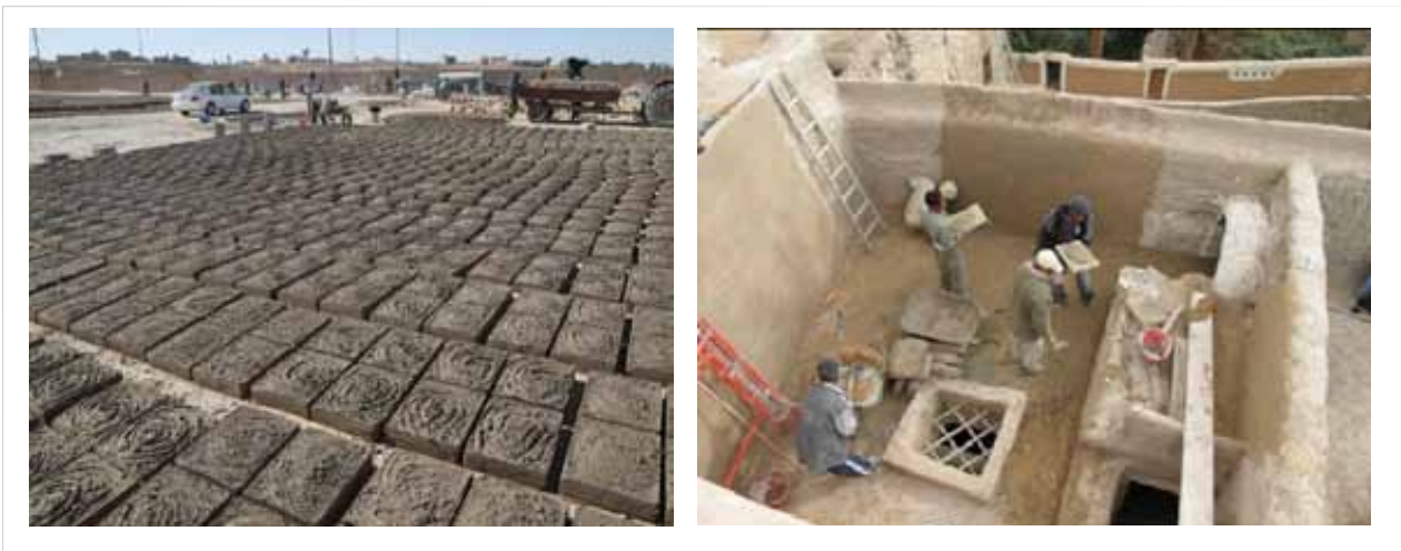
Figure 7: Brick production and restoration works organized in 2009. © Grégoire Paccoud
