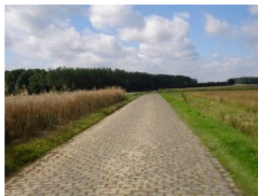
FIGURE 12: CHAUSSEE DE BRUNEHAUT
