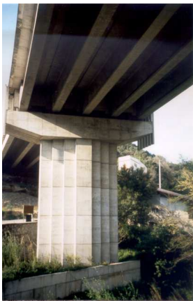
Figure 8: Overall view of a Lodève Bridge pier
