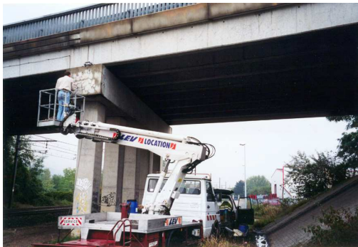
Figure 12: Partial view of the Saint Maurice de Beynost bridge
