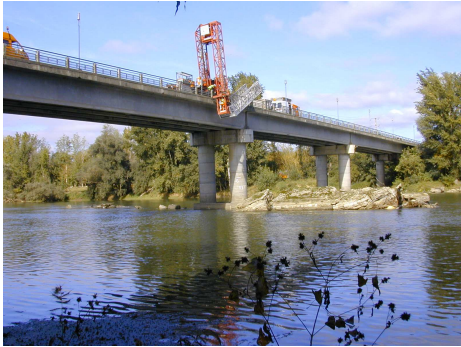
Figure 2: Overall view of the Ondes bridge
