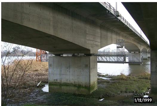
Figure 10: Overall view of The Bellevue Bridge
