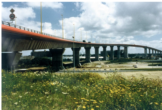
Figure 14: General view of the Cheviré Bridge. (Courtesy G. Forquet)
