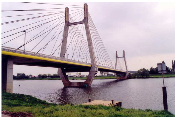
Figure 6: Overall view of the Bourgogne bridge
