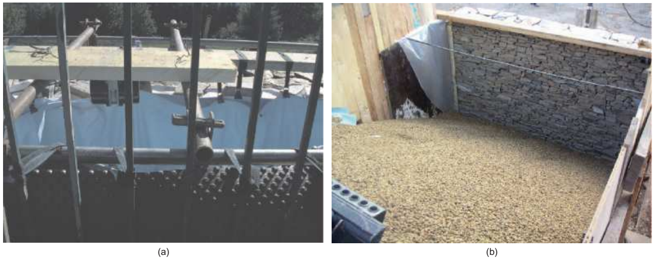
Fig. 5. (a) Hydrostatic loading process; (b) rolled gravel backfill loading process
