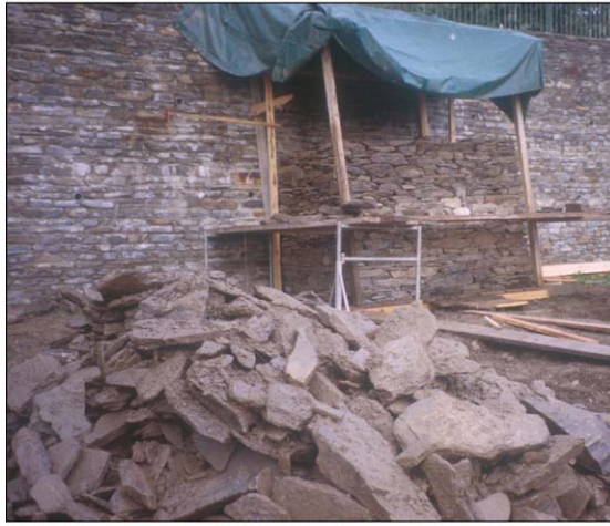
Fig. 5. Wall 5 construction; left: stone size heterogeneity, right: wall basement construction.
