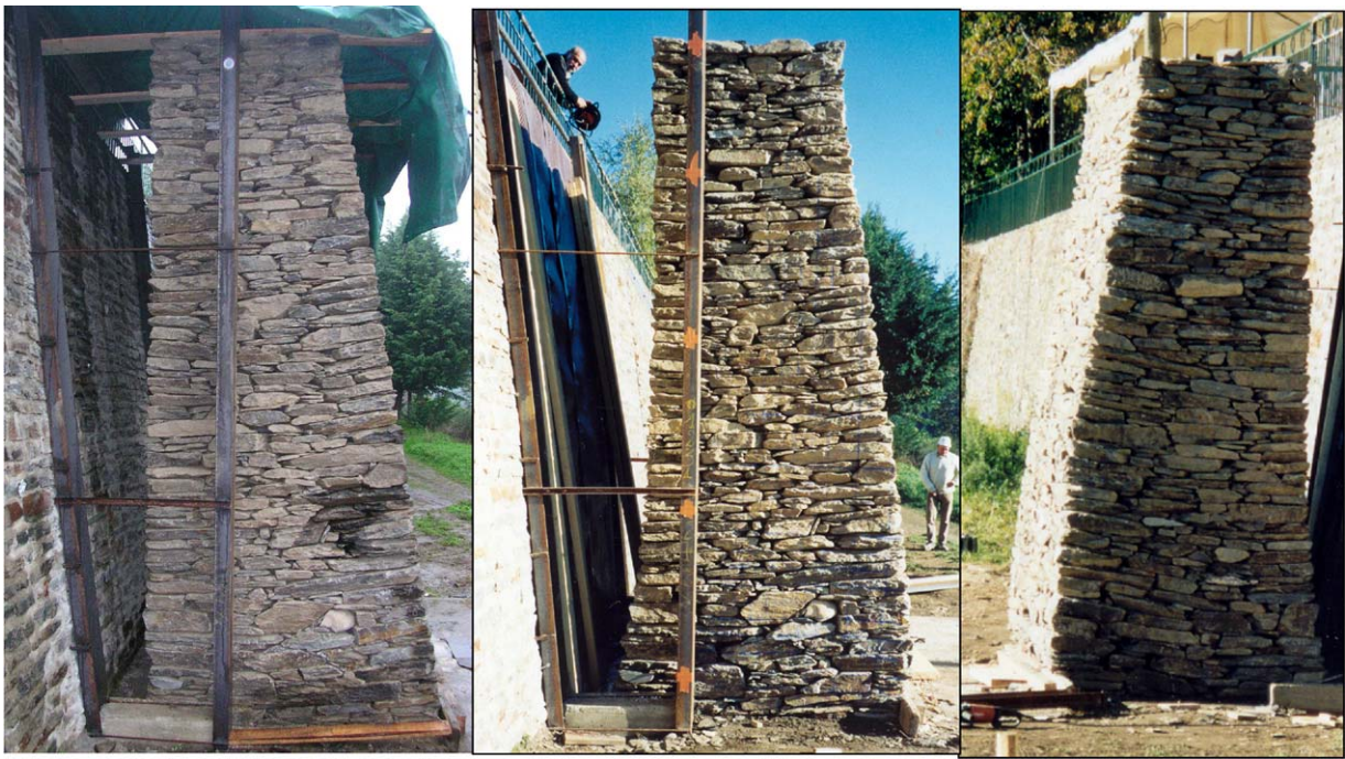
Fig. 7. Wall 5, left: before loading, centre and right: after loading “belly shape”.
