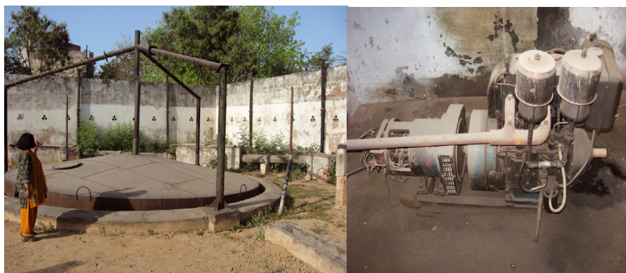
Figure 13. Biogas plant based on community toilet (i.e. human waste) and cow dung for cooking gas and electricity generation.
