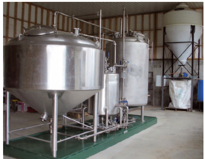
Figure 12b. Stateline Farm in Shaftsbury is gearing up to produce 100,000 gallons per year of biodiesel at its on-farm facility. Photo by Vern Grubinger (www.sare.org).
