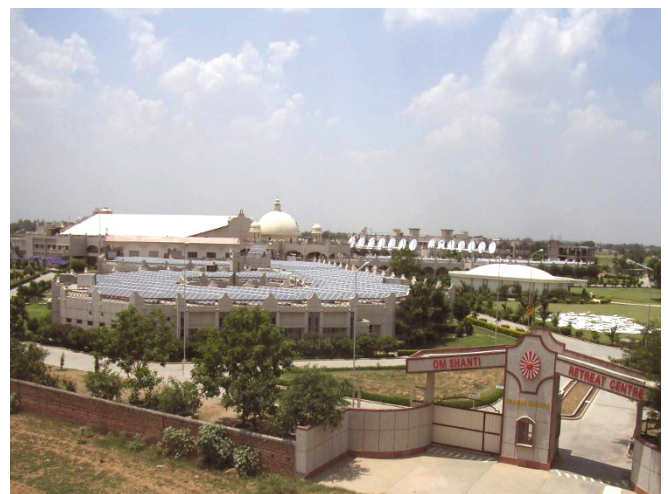
Figure 9b. A 200 kW p solar PV power at the Om Shanti Retreat Center near Delhi (India) (Pilz, 2009).
