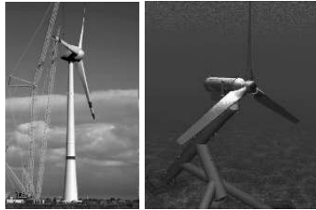
Figure 8.1. The Enercon E126 wind turbine (left) and the Hammerfest Strøm tidal turbine (right) with axial flow
