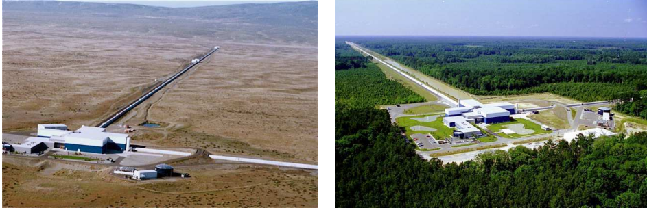
Fig. 27. – Aerial photographs of the LIGO observatories at Hanford, Washington (left) and Livingston, Louisiana (right). The lasers and optics are contained in the white and blue buildings. From the large corner building, evacuated beam tubes extend at right angles for 4 km in each direction which are covered by the arched, concrete enclosures. The full length of only one of the arms is shown in each image. Photos courtesy of the LIGO scientific collaboration.
