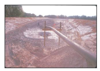
**Figure 3.** Lake-dredged materials being delivered and deposited at temporary containment area.
