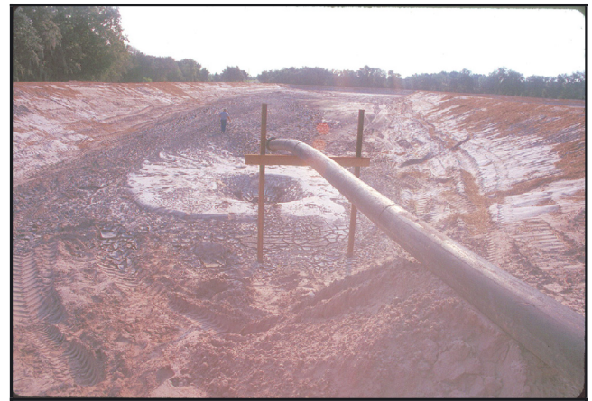
Figure 3. Lake-dredged materials being delivered and deposited at temporary containment area.
