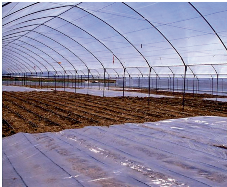
Figure 1. Solarization treatment in the metal-plastic greenhouse.
