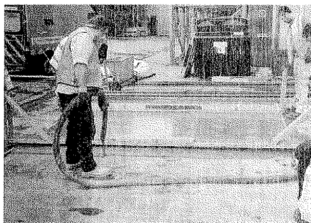
Figure 8. Laying of the mortar
