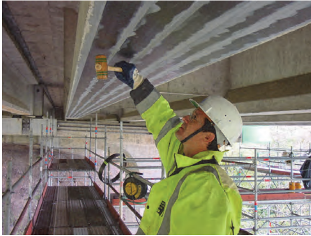
Fig. 1. Inspection with acoustic sounding (hammer tapping).
