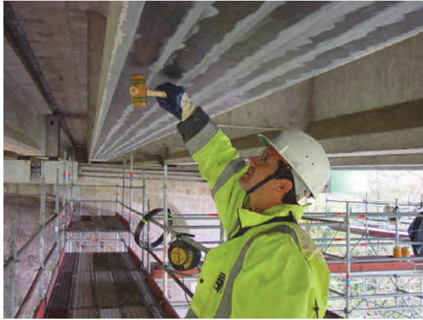
Fig. 1. Inspection with acoustic sounding (hammer tapping).
