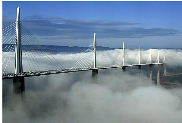
Figure 3: Millau Viaduct – Foster and Virlogeux
