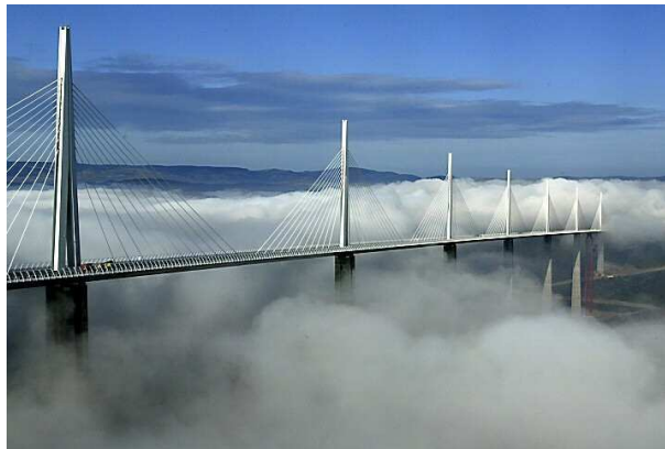
Figure 3: Millau Viaduct – Foster and Virlogeux
