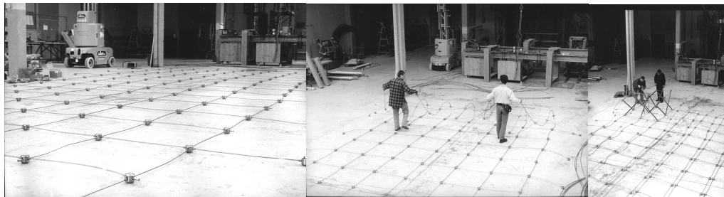
Figure 18: Building the grid
