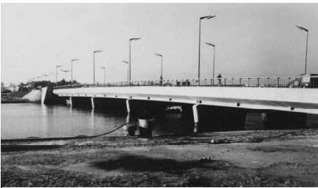
Fig. 12: Houphouët-Boigny bridge. (On the lagoon in Abidjan in Ivory Coast 1954-1957).
