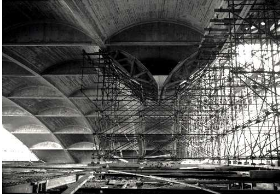
Fig. 16: Removal of the formwork of a wave: the last section of the formwork is tipped out, and interior view of the roofing of a unit on the ground
