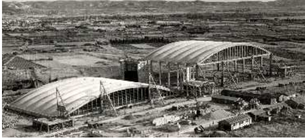
Fig. 15: Marignane Hangars – First par lift – Completed hangars
