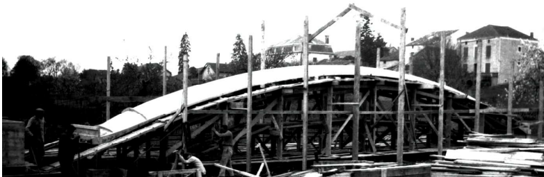
Fig. 14: Marignane Hangars - Formwork for the test wave
