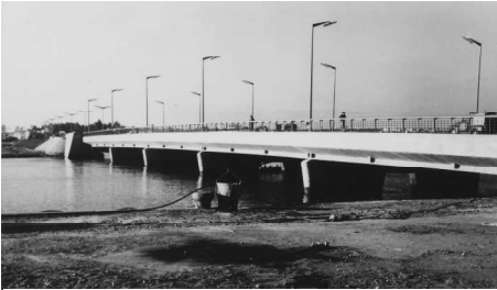
Fig. 12: Houphouët-Boigny bridge. (On the lagoon in Abidjan in Ivory Coast 1954-1957).
