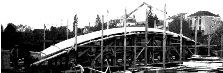
Fig. 14: Marignane Hangars - Formwork for the test wave
