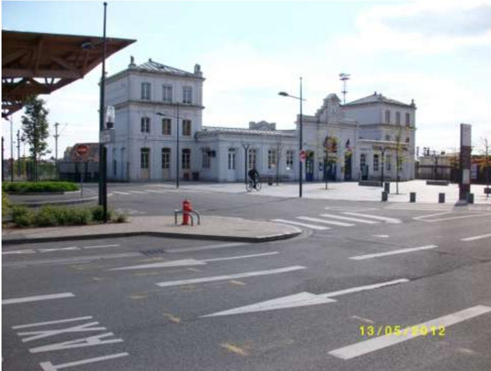
Figure 10 : the legibility of space and functions in the Armentières project (photo L'Hostis-Belibi)
