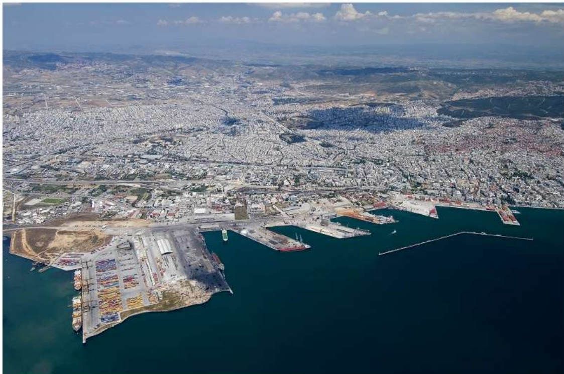
Figure 1. Panoramic view of the central area of Thessaloniki (including port area)
