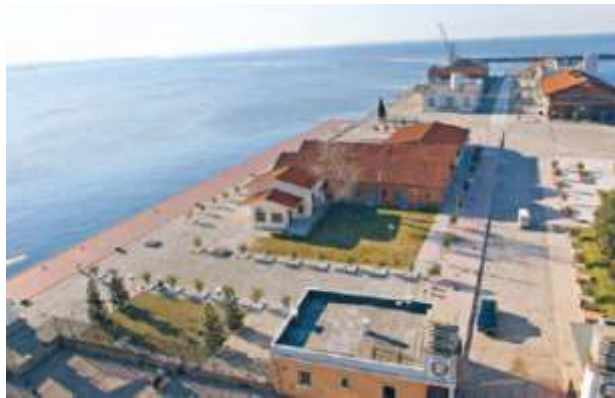
Figure 16. Aerial view of pier no1.
