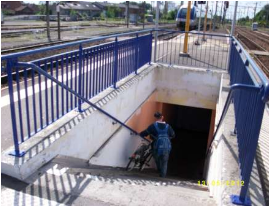
Figure 13 : bicycle rail on the side of the stairs to the platform in Armentières (photo L'Hostis-Belibi)
