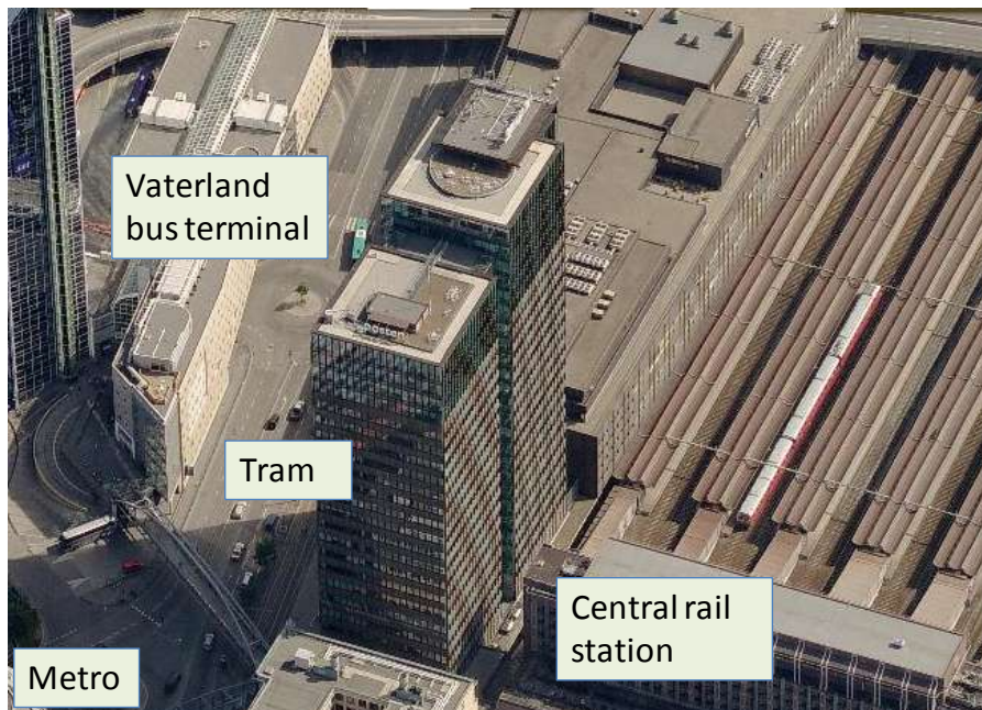
Figure 7. Overview of Vaterland bus terminal
