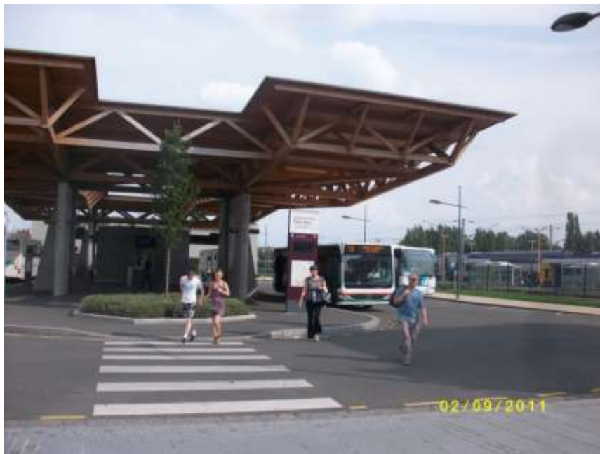
Figure 12 : Armentières bus terminal, an aesthetic design with functional shortcomings (photo L'Hostis-Belibi)
