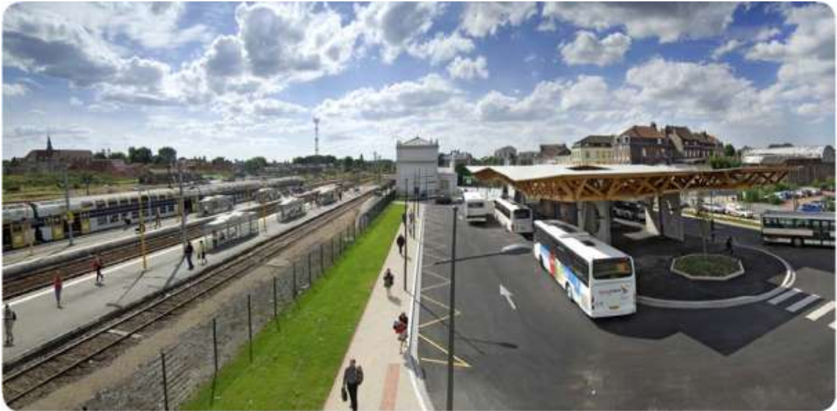
Figure 6: General view of the Armentières exchange pole (source PDU 2010)
