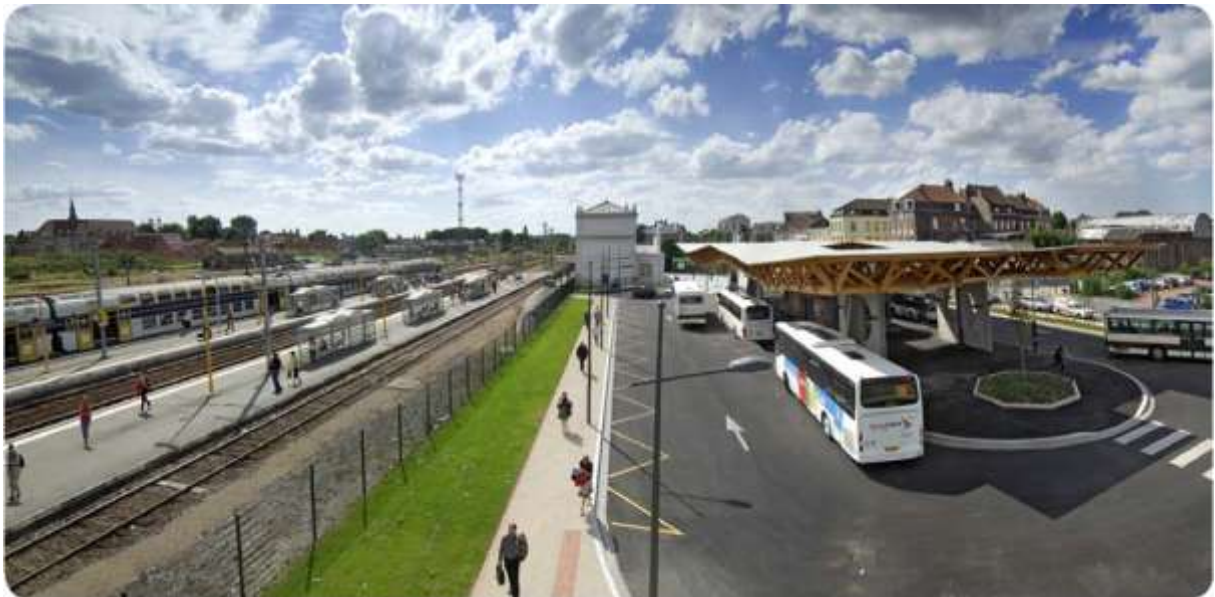
Figure 1 : general view of the Armentières exchange pole (source PDU 2010)
