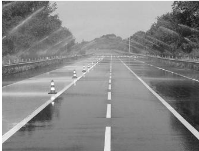
Figure 8 - Ifsttar test track sprinkling system
