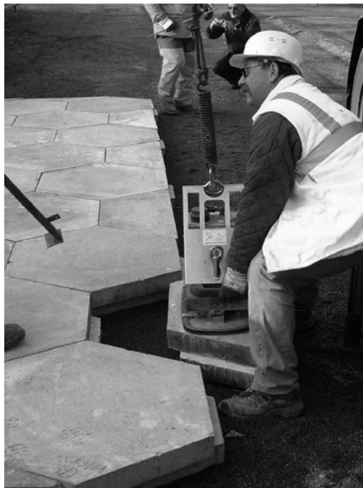
Figure 8: The Autun solution (slabs with connection keys)
