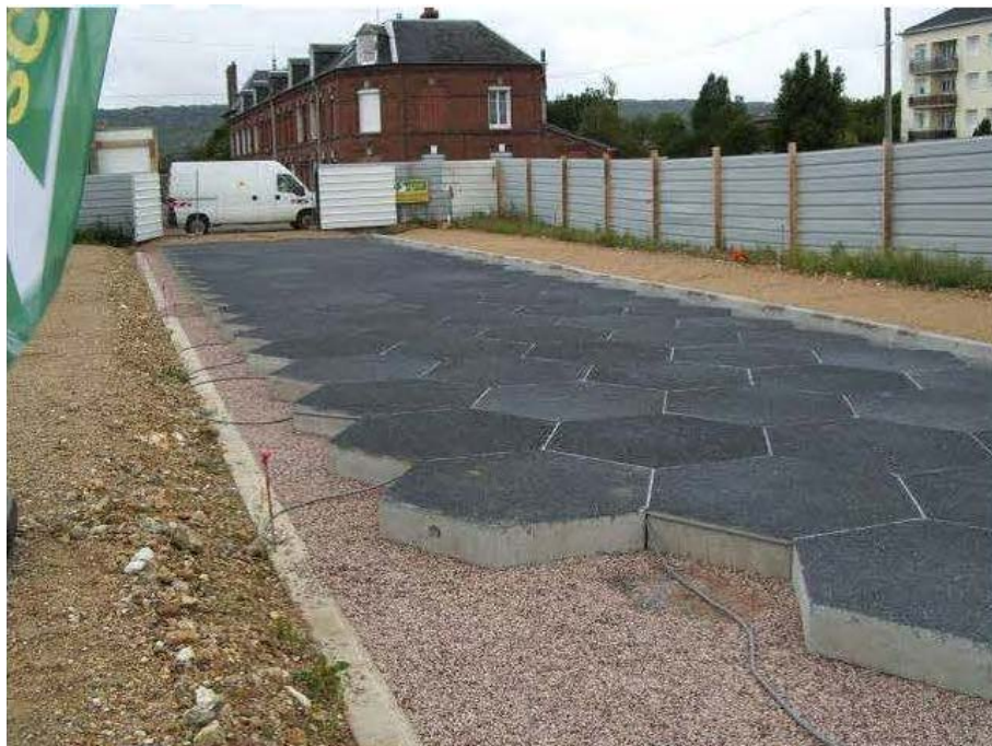
Figure 6: Construction of the Saint Aubin RUP
