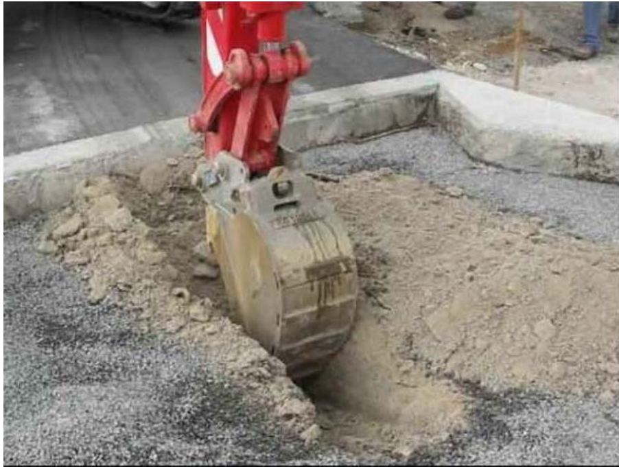
Figure 2: Excavation of the SECTM base course
