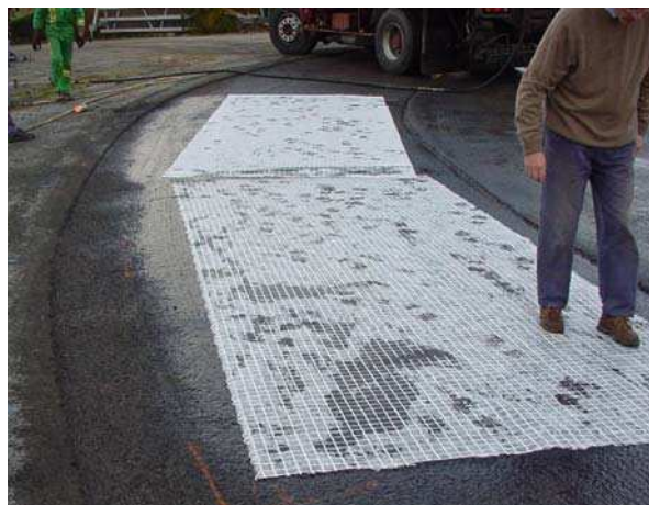
Figure 8. Geogrid after tack coat application on the structure
