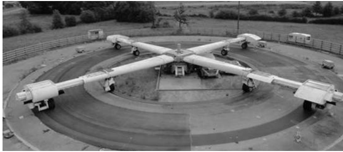
Figure 1. View of the IFSTTAR pavement testing facility
