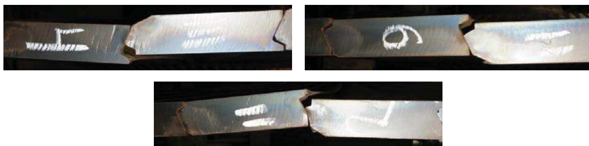
Figure 1. The damaged detachable shrouds of the steam turbine blading after the 3 years of operation (the series of temperature overloading was missed in operation of the turbine)
