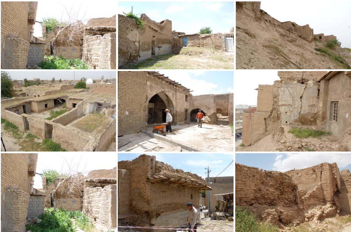
Partially collapsed structures
