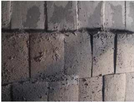
FIGURE 1. New (top) and old (bottom) SiC based refractory tiles in a WTE facility (tile height: 245mm)
