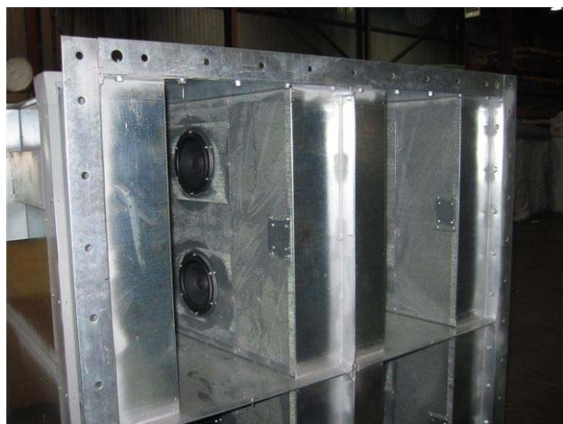
Image 13: Active Noise Attenuator Showing Speakers
