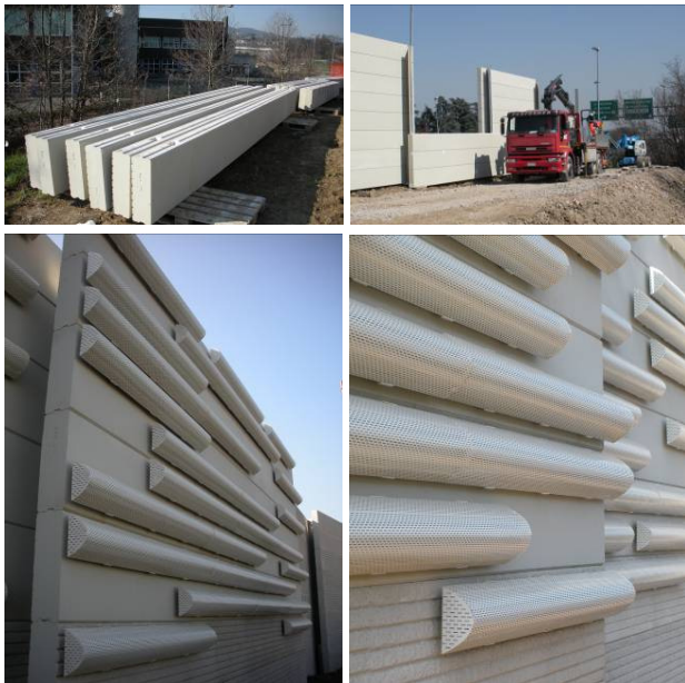
Figure 2: some pictures of analyzed noise barriers: panels made by autoclaved aerated concrete before the assembly (upper left side), operations of in situ assembly of the panels (upper right side), noise barrier with semi-cylindrical acoustical absorbers (bottom left side), detail of acoustical absorbers (bottom right side).
