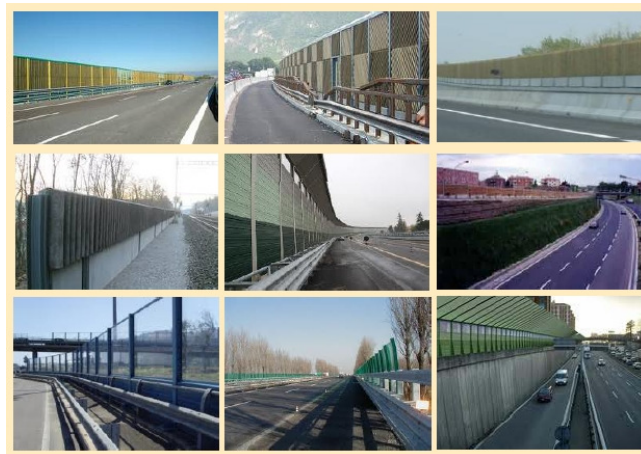
Figure 1: examples of noise barriers installed on the sides of highway infrastructures.
