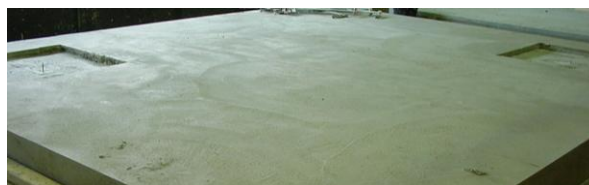
Figure 1: Concrete test floor (180mm in thickness)
