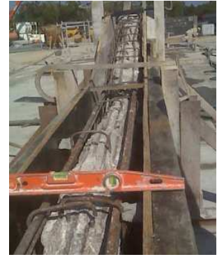
Figure 4. Repair techniques: (a) beam after hydrodemolition, (b) wet/dry shotcrete(c) formed concrete.
