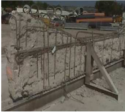
Figure 4. Repair techniques: (a) beam after hydrodemolition, (b) wet/dry shotcrete(c) formed concrete.
