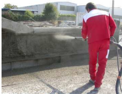
Figure 4. Repair techniques: (a) beam after hydrodemolition, (b) wet/dry shotcrete(c) formed concrete.
