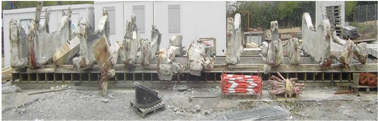
Figure 5. Beams after 80 years of exposure.
