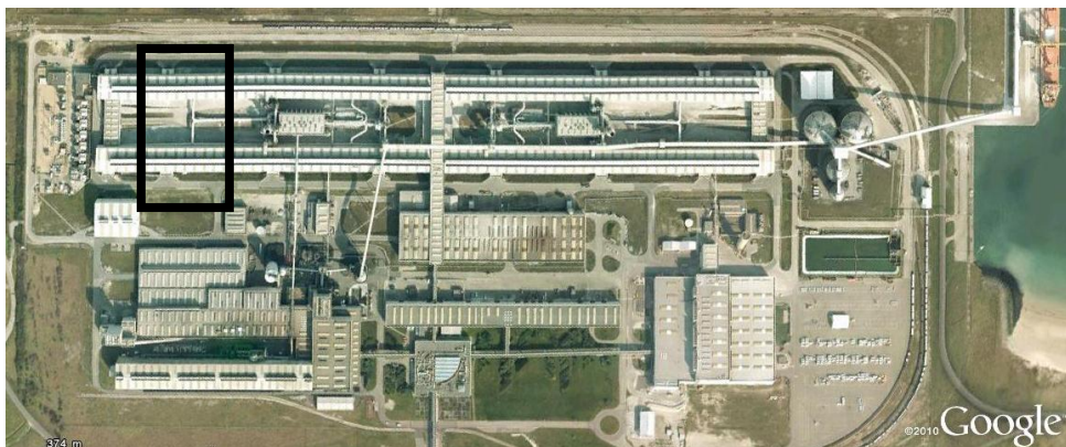
Figure 2. Aluminium Dunkerque, France (©2010 Google). The substation is surrounded by a rectangle.
