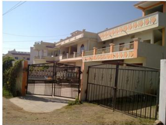
Photo 4.4: Pucca Houses in Deepdi Abadi Area
