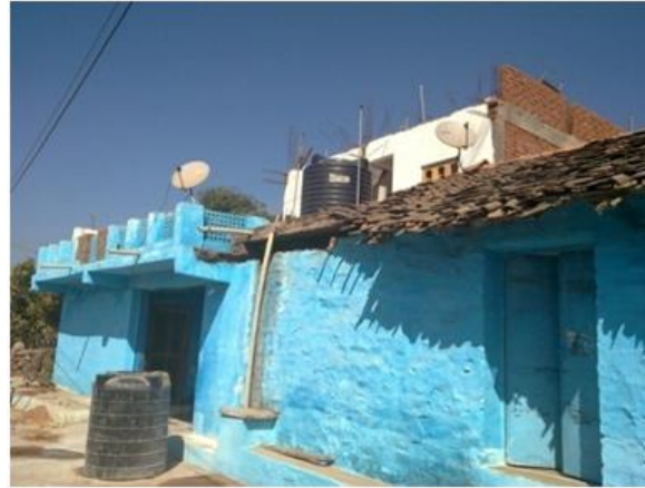
Photo 4.14: DTH Service in Semi-pucca houses in Barkheda Salem Village
