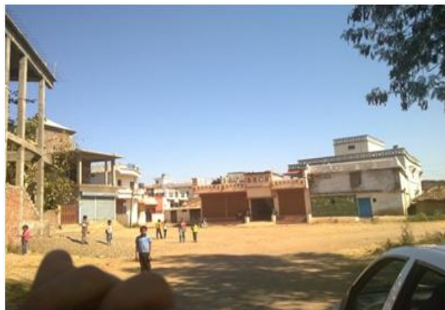
Photo 4.12: Pucca buildings in Abadi Area of Mugaliya Chhap Village
