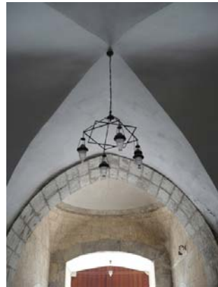
(pic. 20) Belen. Sultan Süleyman caravanserai, vestibule with cupola and groin vault of hall. 2008
