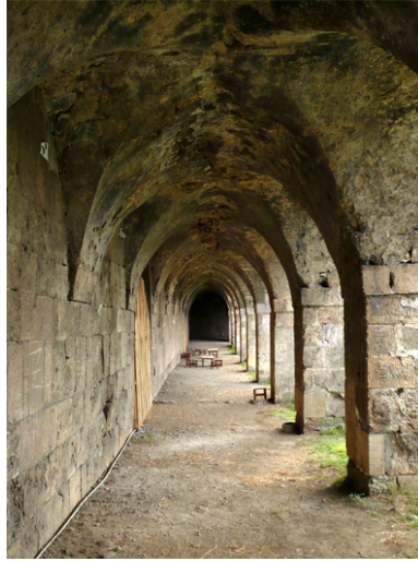
(pic. 14) Payas. Sokullu Mehmet Paşa caravanserai, court arcade with groin vaults. 2008
