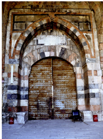
(pic. 12) Payas. Caravanserai portal on bazaar street. 2008.
