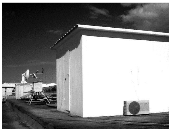
Fig 5 : Vue of the Test cell and the outdoor unit of the split-system.
