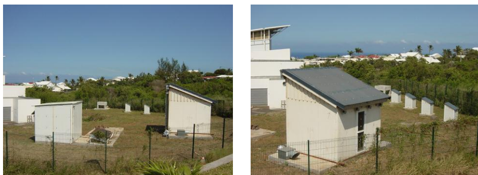
Fig 6 & 7. The experimental platform and the test cells
