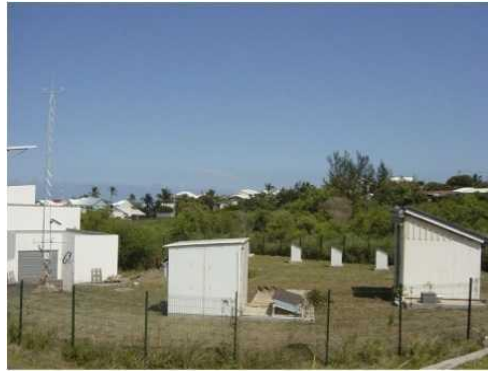
Figure 5. Experimental site for L.P.B.S. Laboratory
