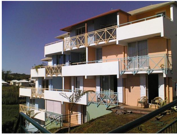
Fig. 8 : The final project (april 1999)
