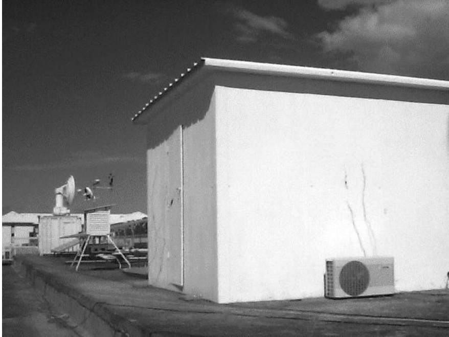
Fig. 2. Picture of the test cell seen from North-West
