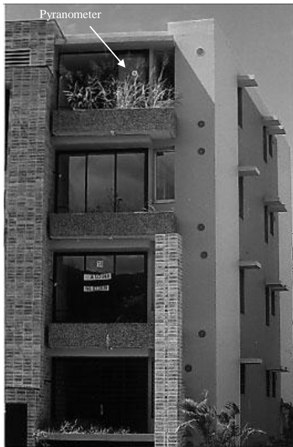
Fig.6 : Experimented dwelling on its last floor (West side)
